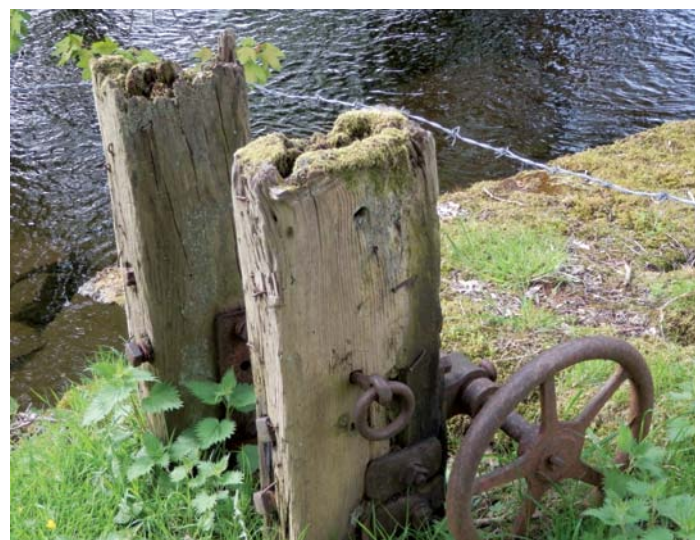
Remains of weir machinery
